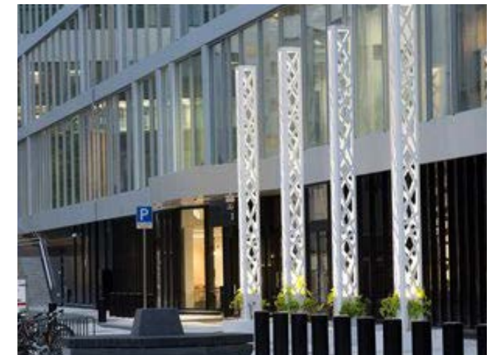
Lighting integrated into wayfinding structures.
