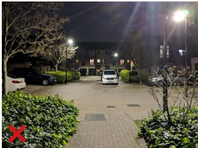
Cluttered, poorly located lighting increases the risk of vehicle strikes
