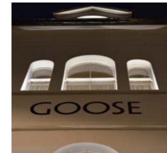
Close offset lighting reduces spill
