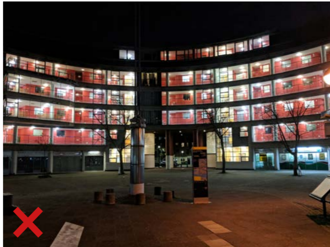
Unsympathetic soffit mounted lighting to walkways creates glare and spill light
