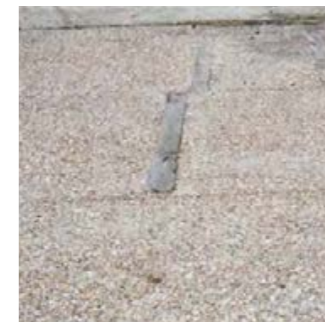
In-situ exposed aggregate concrete slabs with timber lengths set-in Vary movement joint grid and arrangement of timbers dependent on location.
