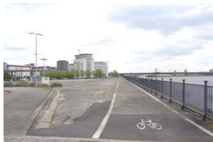
Metal railings to Royal Victoria Dock
