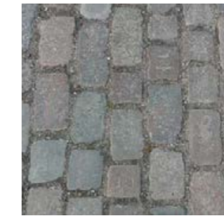
Granite setts To be used as tactile edge to paths, or other edge detail. Not to be used within path routes to ensure accessibility.
