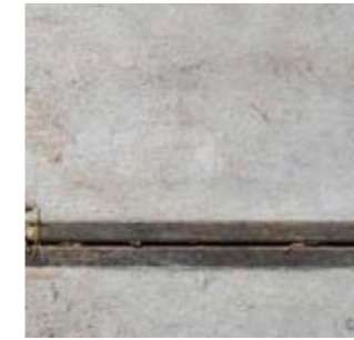
Stelcon pre-cast smooth concrete slabs with steel cornering To be used on or off-plot, and specifically on the dock edge. Ensure there is requisite depth for product, especially in areas of false quay.
