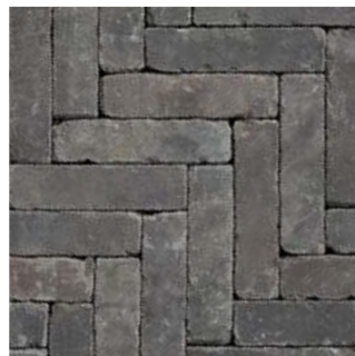
Clay paviors On and off-plot use - vary movement joint grid depending on location.
