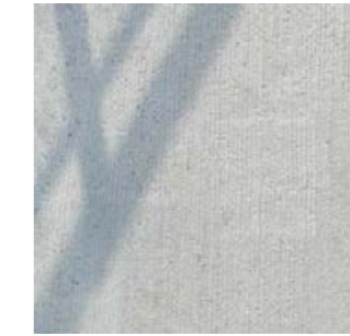
In-situ brushed concrete slabs On and off-plot use - vary movement joint grid depending on location.
