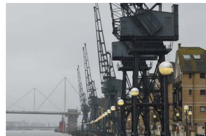
Shipping cranes - Royal Victoria Dock
