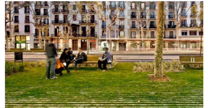
In-situ exposed aggregate concrete slabs with timber lengths set-in Vary movement joint grid and arrangement of timbers dependent on location.
