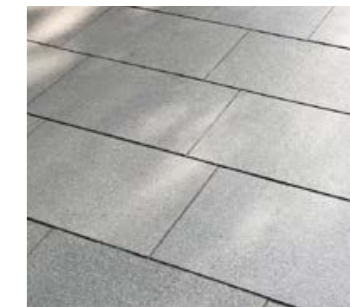
Granite paving slabs To be used where more formal hard surfacing is desired.
