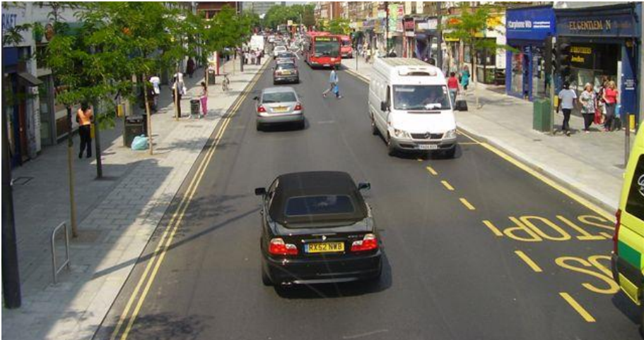
Walworth Road, Southwark. A good example of how road narrowing can contribute to traffic calming, as well as creating generous pavement widths that can support tree planting, cycle parking and other improvements.
